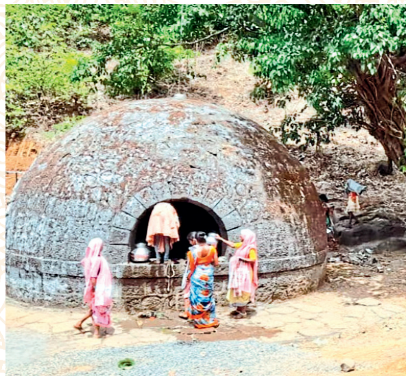
Well in Kasara Ghat
