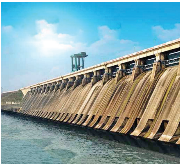
A representative photograph of Hirakund Project, Odisha
